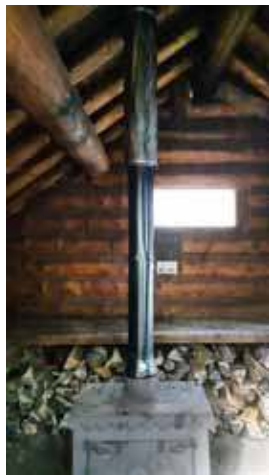
New stove pipe
